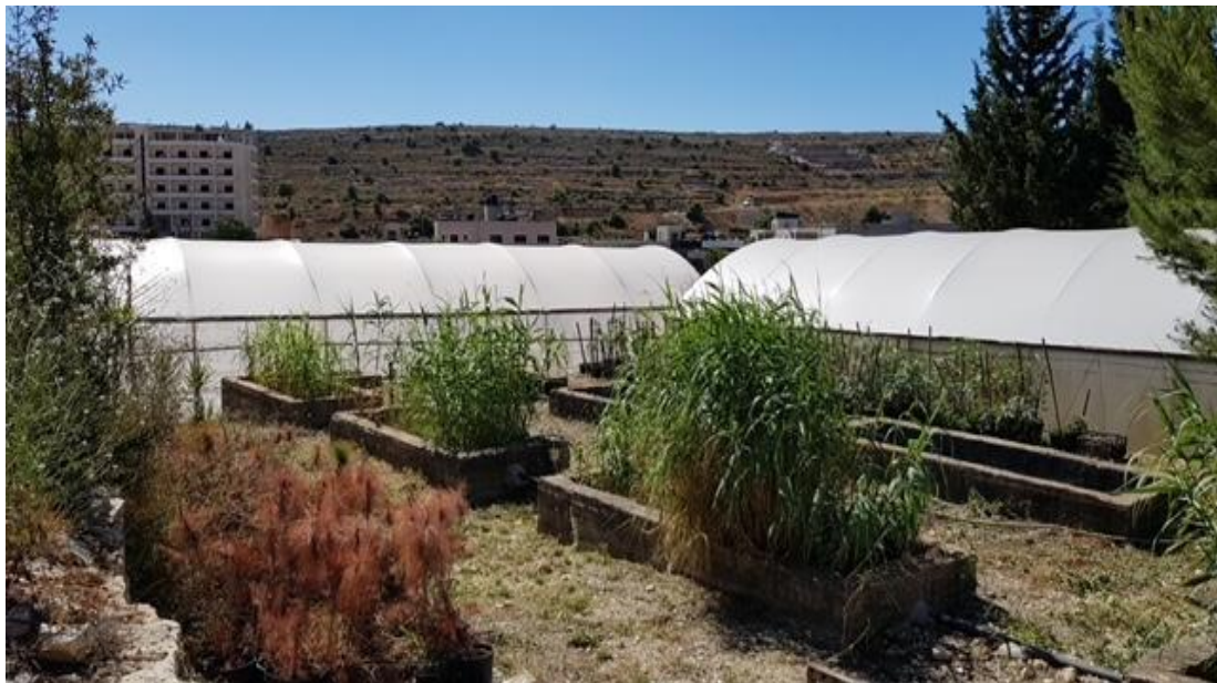
Last three beds of the four beds in series of the pilot CWs installed at Birzeit University
