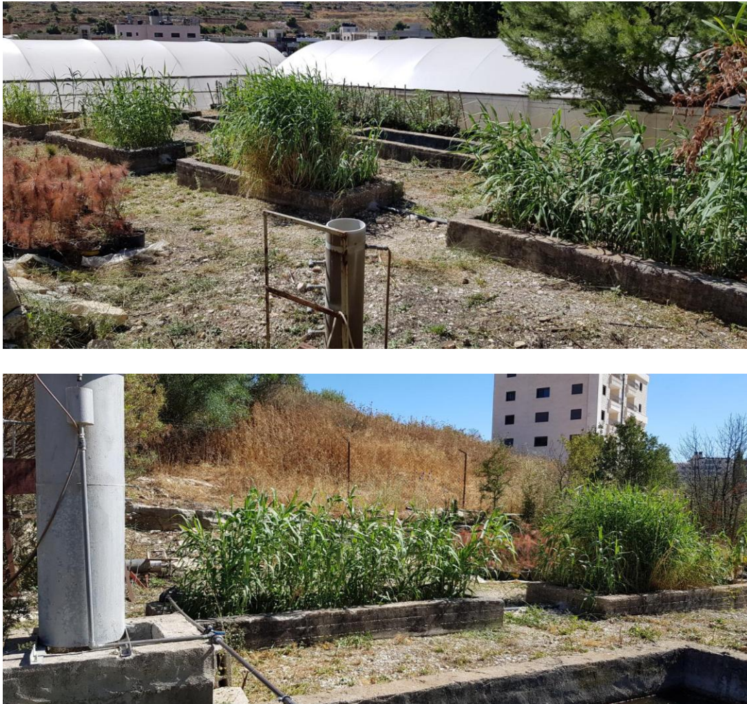
Fig (6): Pilot system of constructed wetlands at Birzeit University campus
