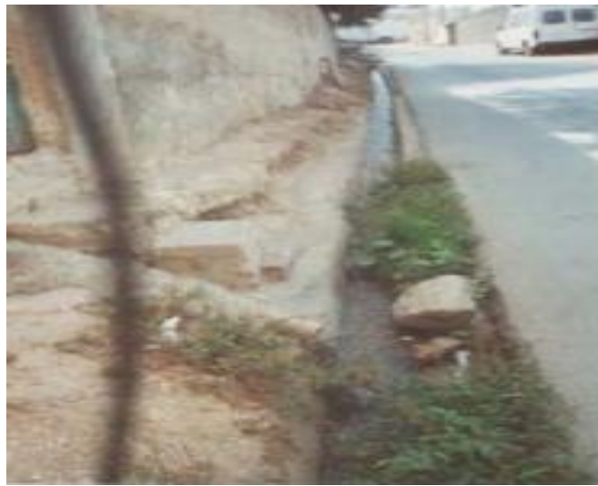
Photo 1: Sewerage pipe replacing open channel in Jalazoun Refugee Camp (Mahmoud et al., 2008).
