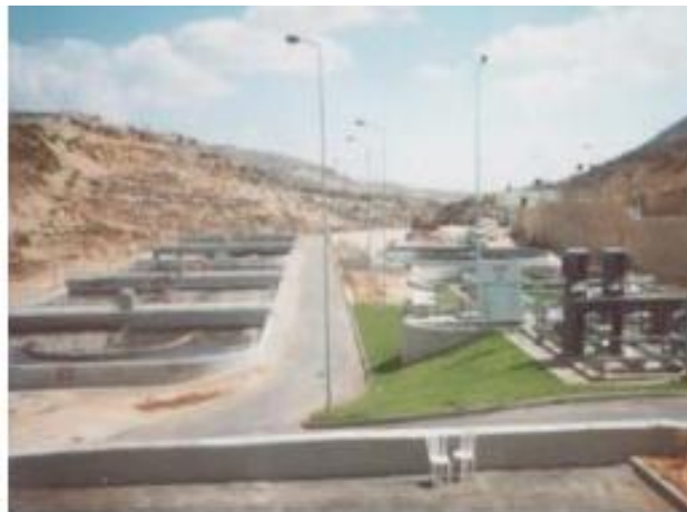
Photo 5: Al-Bireh extended aeration system for wastewater treatment
