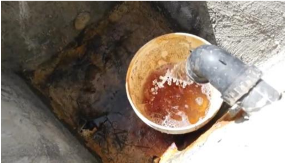
Final outlet from the constructed wetlands
