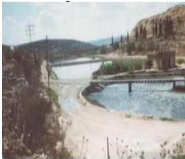
Photo 3: Ramallah oxidation pond system for municipal wastewater treatment
